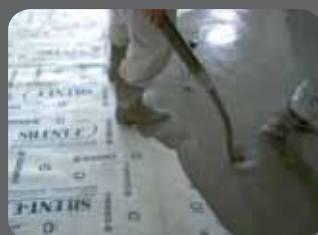
6. Cast the regulation slab
