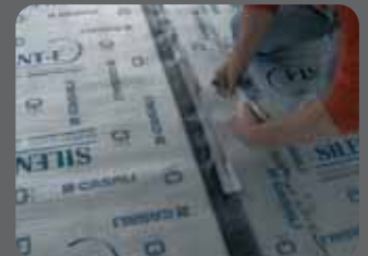
4. Stabilize the membrane by taping the joints
